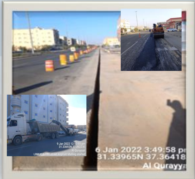
Micro trench & Milling and paving
