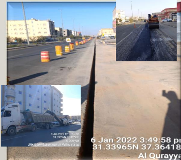
Micro trench & Milling and paving
